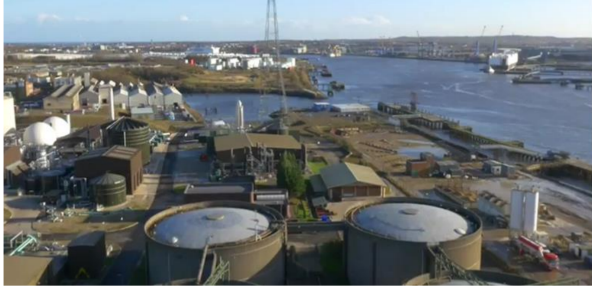
Figure 1 – Aerial Photograph of sludge processing area of Tyneside Wastewater Treatment Facility, Newcastle
